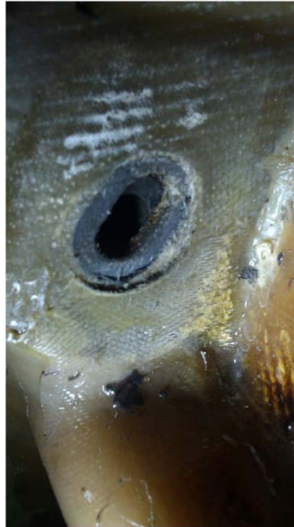
Figure 1 – Showing inspection Side view. (See Figure 2 for Top)
