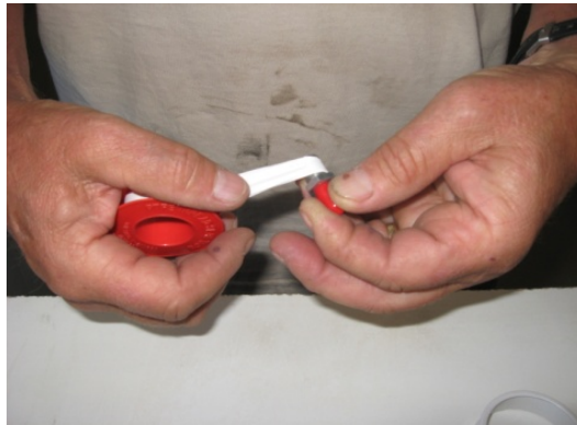
FIGURE 32-40-10-01-c Apply Teflon tape or pipe thread dope to fitting thread
