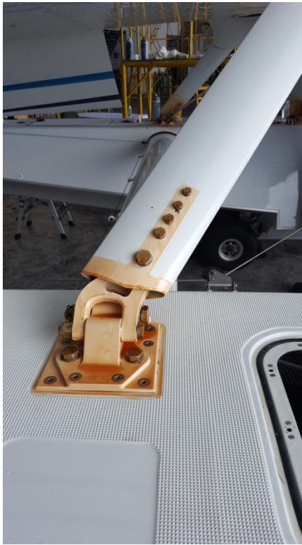
Plate 5: Tape Removed Showing Clean Lines
