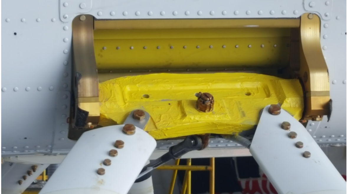
Plate 3: Trunnion Sprayed with ARDROX AV 30™ (Fairing removed)
